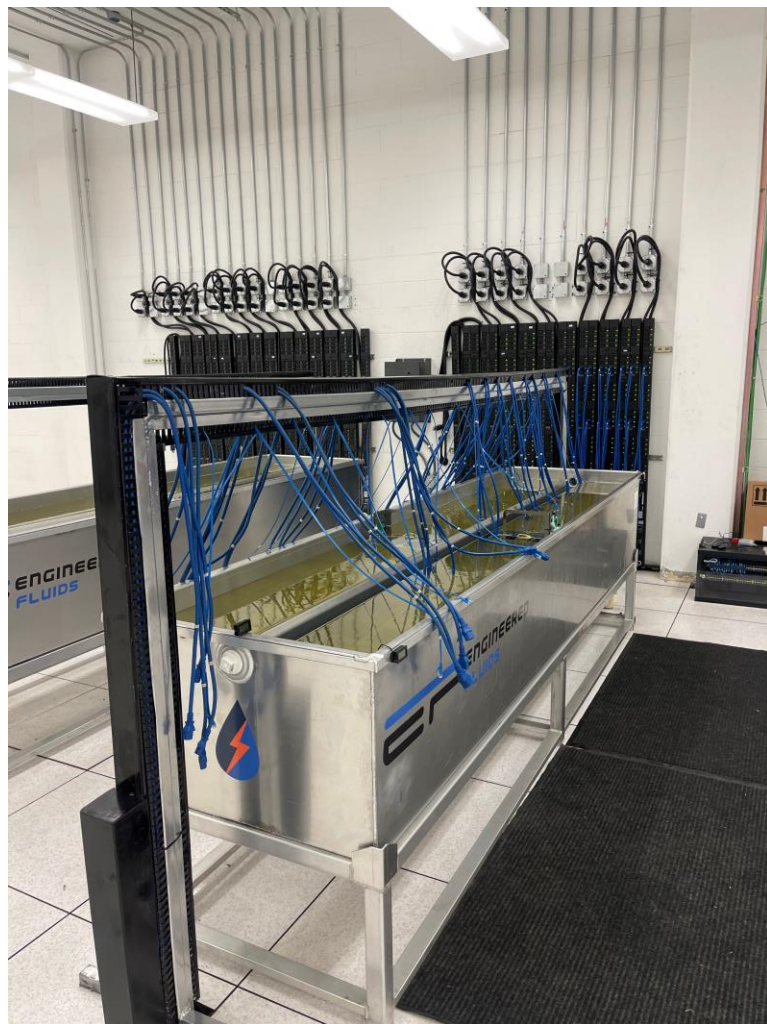
2x SLICTank Module – 675kW Total Module Capacity
